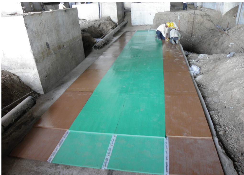
Installation of the green Sylomer layer at the Salaya plant in Gujarat. The structural column of the turbine generator building is near the VIS (left).
